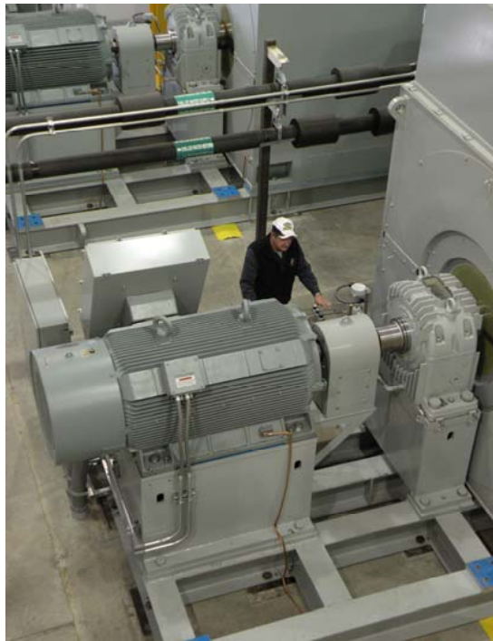
Synchronous Condensers
