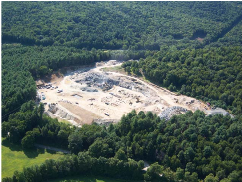
New 345kV Substation Being Constructed in Former Gravel Pit
